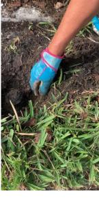
Shown Above: (L) Using a sod cutter to clear away the sod at the sprinkler head location, (R) removing the sod from around the sprinkler head by hand.
